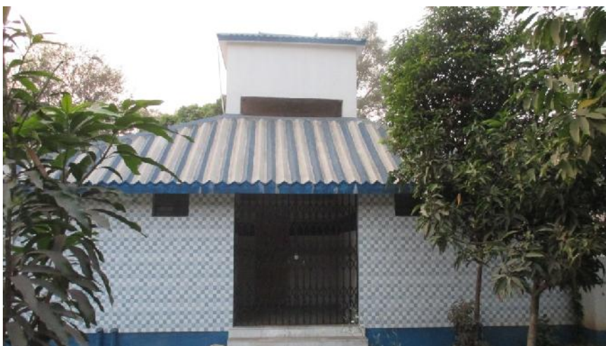
Photo: - Community Latrine
