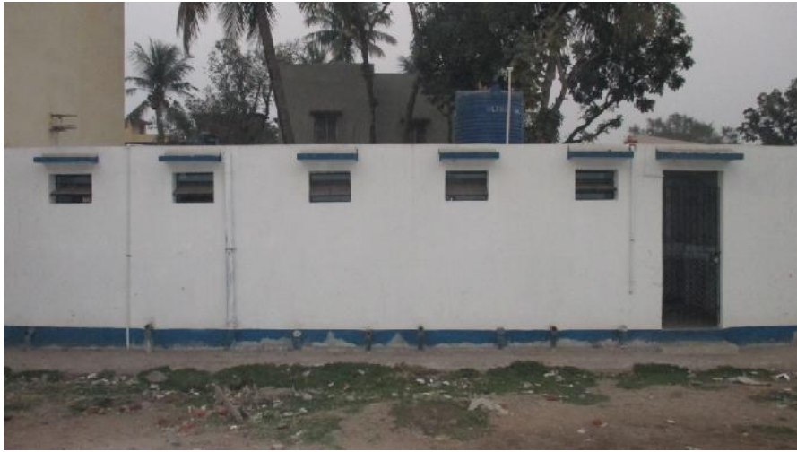
Photo: - Community Latrine
