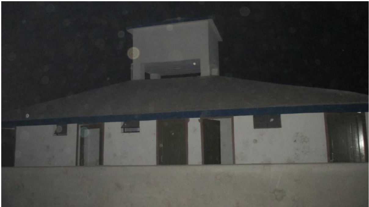
Photo: - Community Latrine
